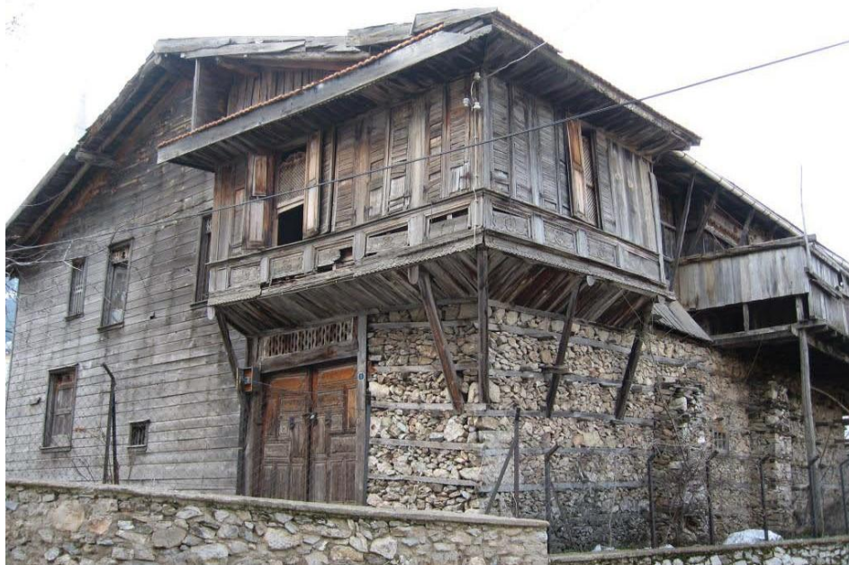
Fig. 4: Municipality Guest House in Ormana (İbradı) , southeast façade, (Çelik, 2009)
