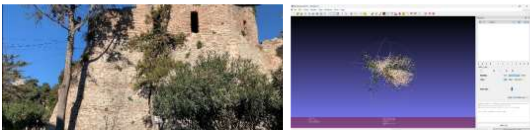
Figure 18 Figures showing the real construction of the surrounding walls and the generated point cloud of it in MeshLab
