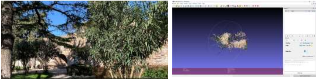
Figure 19 Figures showing the real construction of an arched wall and the generated point cloud of it in MeshLab
