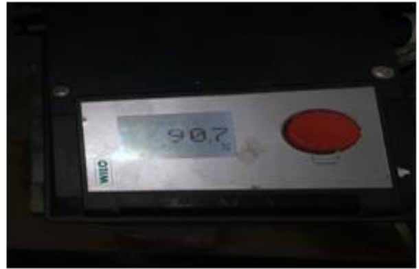
Figure 22. PLC mounted on the system. As you can see in 7.6 Bar with the SET POINT 7.5 only one motor is working with 90% of the power when the pressure drops to 5.0 the motor one reaches the maximum and the second motor starts working.
