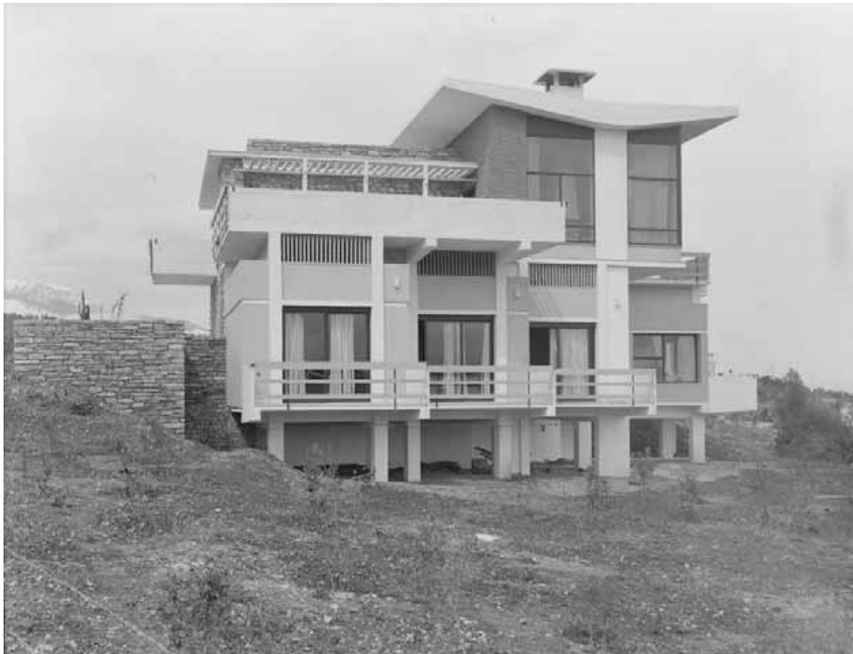
Fig. 8: Ph. Vokos, Xenia Highway Station with accommodation at Platamonas (Source: Benaki Museum Photographic Archives)
