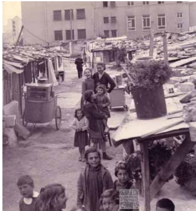
Fig. 2: Sheds in Athens in the 50s (Source: Modern Social History Archive)
