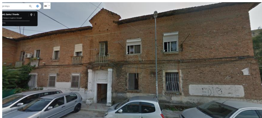
Figure 11. Selected Building located in Tirana City Façade 1
