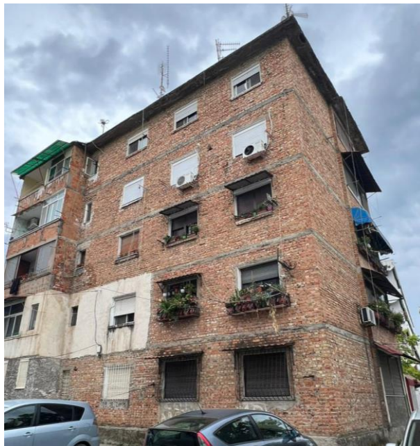
Figure 8. Rectangular opening in masonry walls in Tirana, Albania
