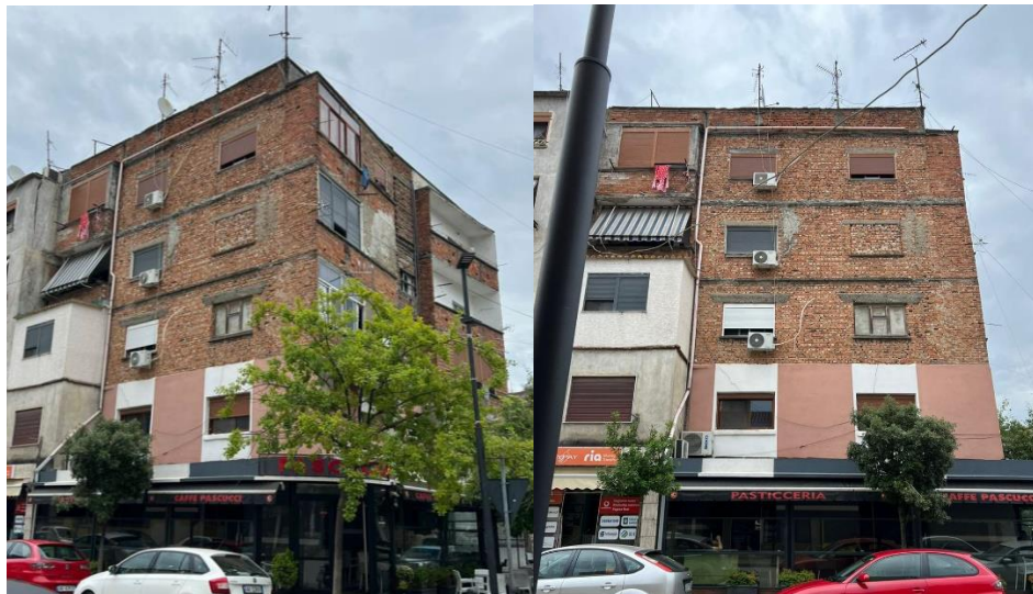
Figure 1. Unreinforced masonry walls with openings in Tirana, Albania
