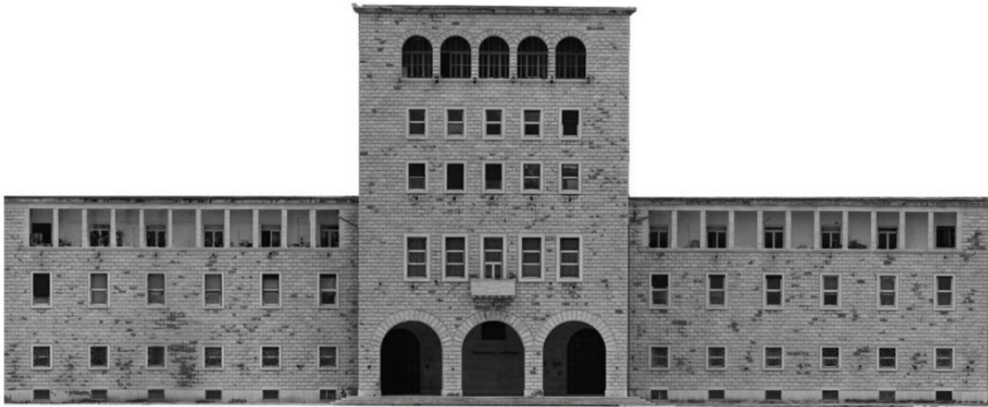
Figure 20. An architectural survey of the facade is conducted within the framework of investigating pathologies, analyzing the distribution of cracks, and identifying fractures.
