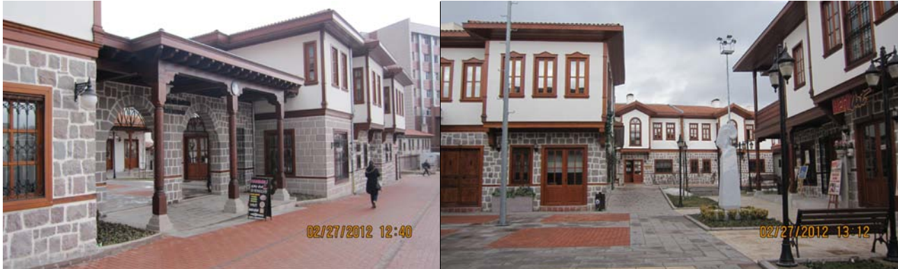
Figure 3, Hamamonu district structure after rehabilitation project
