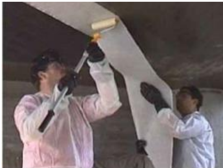
Figure 37. The placement of carbon fibers.
