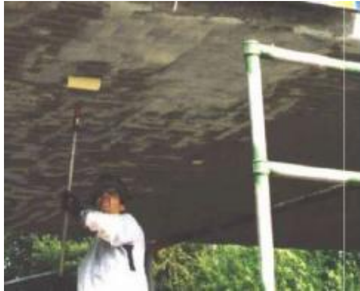
Figure 36. The application of primer according to the manufacturer's specifications,
