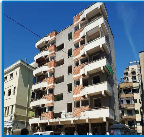
Figure 15. Vip RC frame buildings in Durrës
