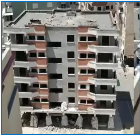
Figure 17. Vip building – CT demolition
