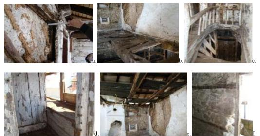
Fig. 3: a. Damagedinternal wall constructed by clay reinforced with timer willows; b. c. & e. deterioration of a timber elements at ceiling/flooring and staircase structure; d. pour maintenance of planking envelope; f. misapplied of structural conservation.
