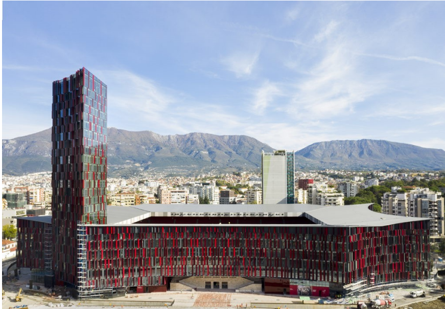
Figure 9. Air Albania Stadium
