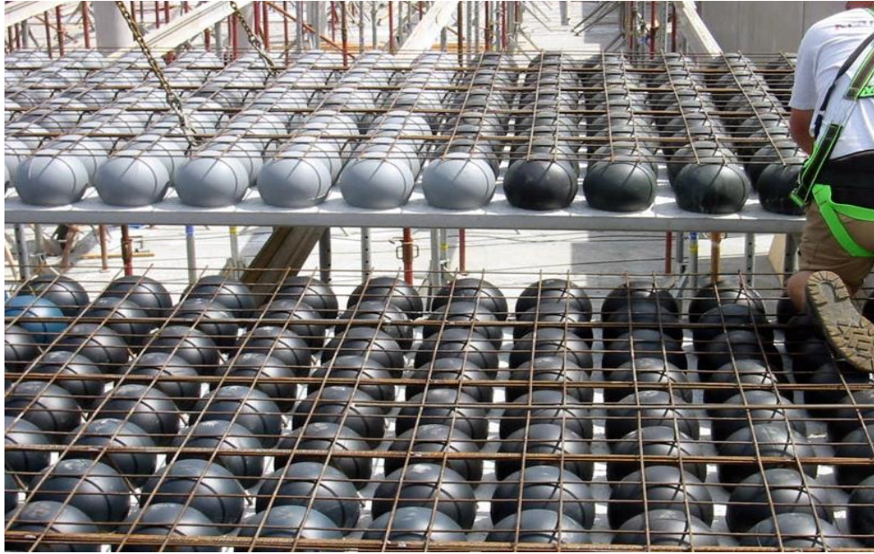
Figure 6 Different size of Cobiax balls (Zielstattstrasse 27)
