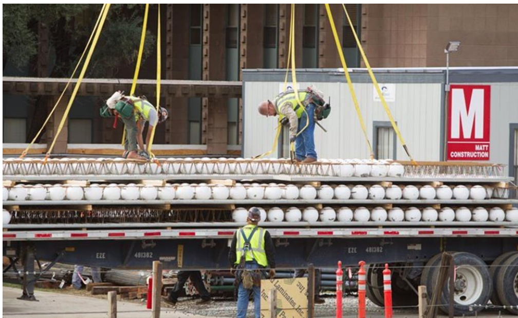
Figure 5 Transportation of Cobiax from factory to site
