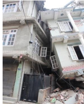
Figure 40. Collapse of buildings results in pounding in adjacent buildings in Chautara, Sindhupalchowk.
