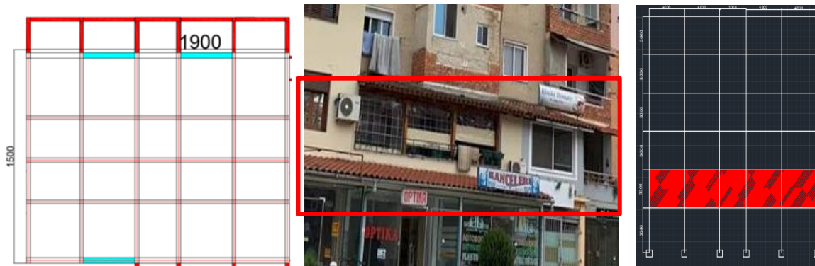
Fig 68. second floor overhangs due to human intervention by adding extra rooms.
