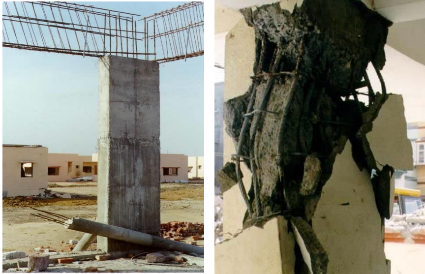
Figure 46. A Zoom+ view of building in on-going construction with not proper reinforcement detailing for Beam-Column joint.
