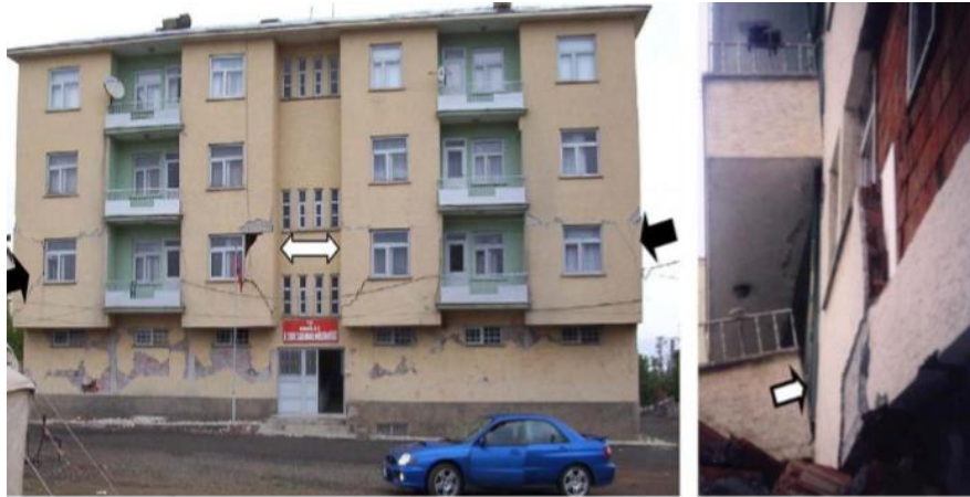
Fig 37. Failure due to overhangs [Dog˘angu˘n 2004]
