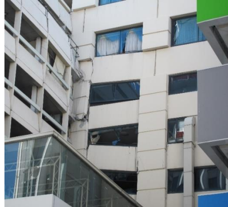
Figure 39. Buildings Pounding Damages Observed in the 2011 Christchurch earthquake Christchurch Earthquake.
