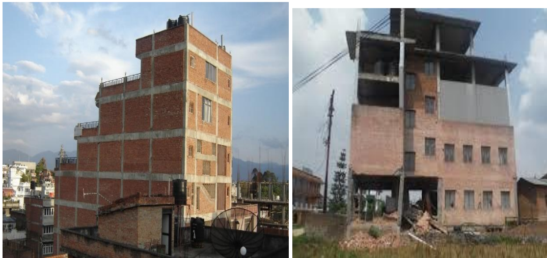
Figure 19. Stepped RC building with masonry infill. [Yukta Bilas Marhatta, Nepal].
