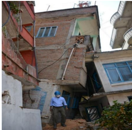
Figure 40. Collapse of buildings results in pounding in adjacent buildings in Chautara, Sindhupalchowk.
