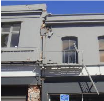
Figure 39. Buildings Pounding Damages Observed in the 2011 Christchurch earthquake Christchurch Earthquake.
