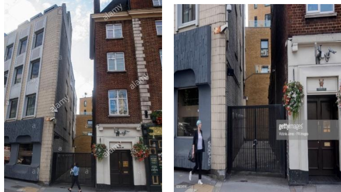
Figure 42. The three-metre gap between two buildings on Euston Road in central London.
