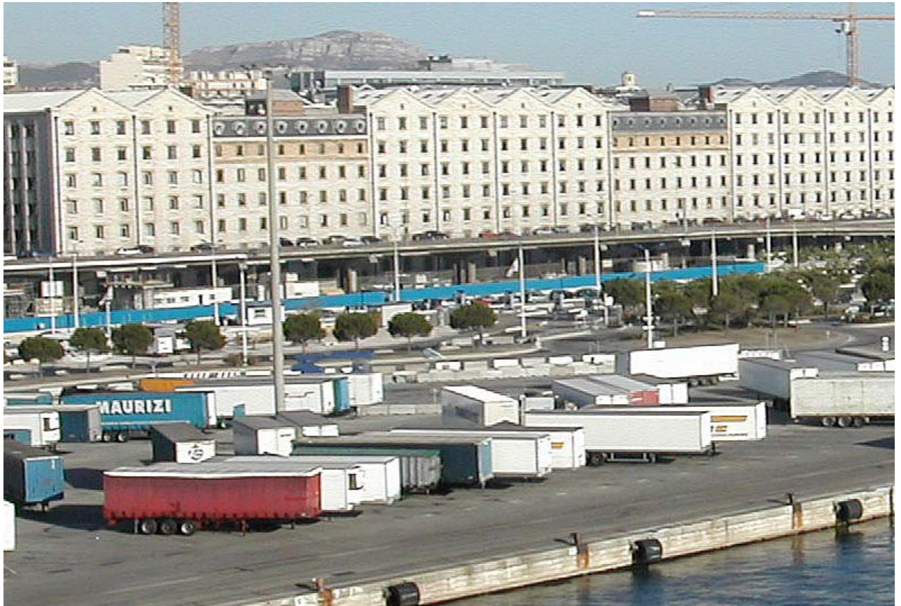
Fig.5 The renovated Docks of Marseille (Aix-Marseille, 2007)
