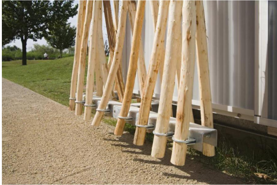
Figure 17. Detail of wood structure used for the facade, (ArchDaily,2009)
