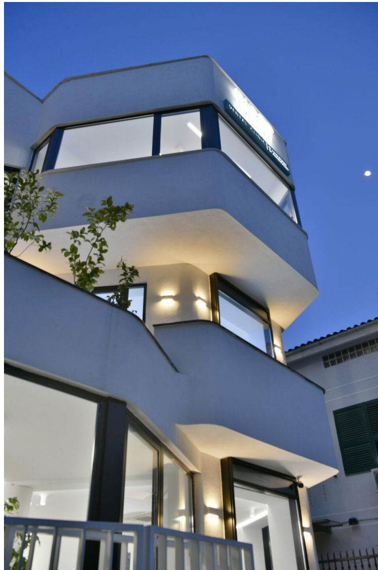
Figure 34. The northeast openings of the clinic. (By author)
