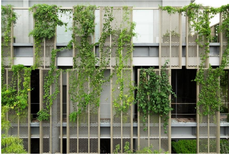
Figure 164. Residential complex in Shanghai using green facade Shang Kai Steel's SKA.
