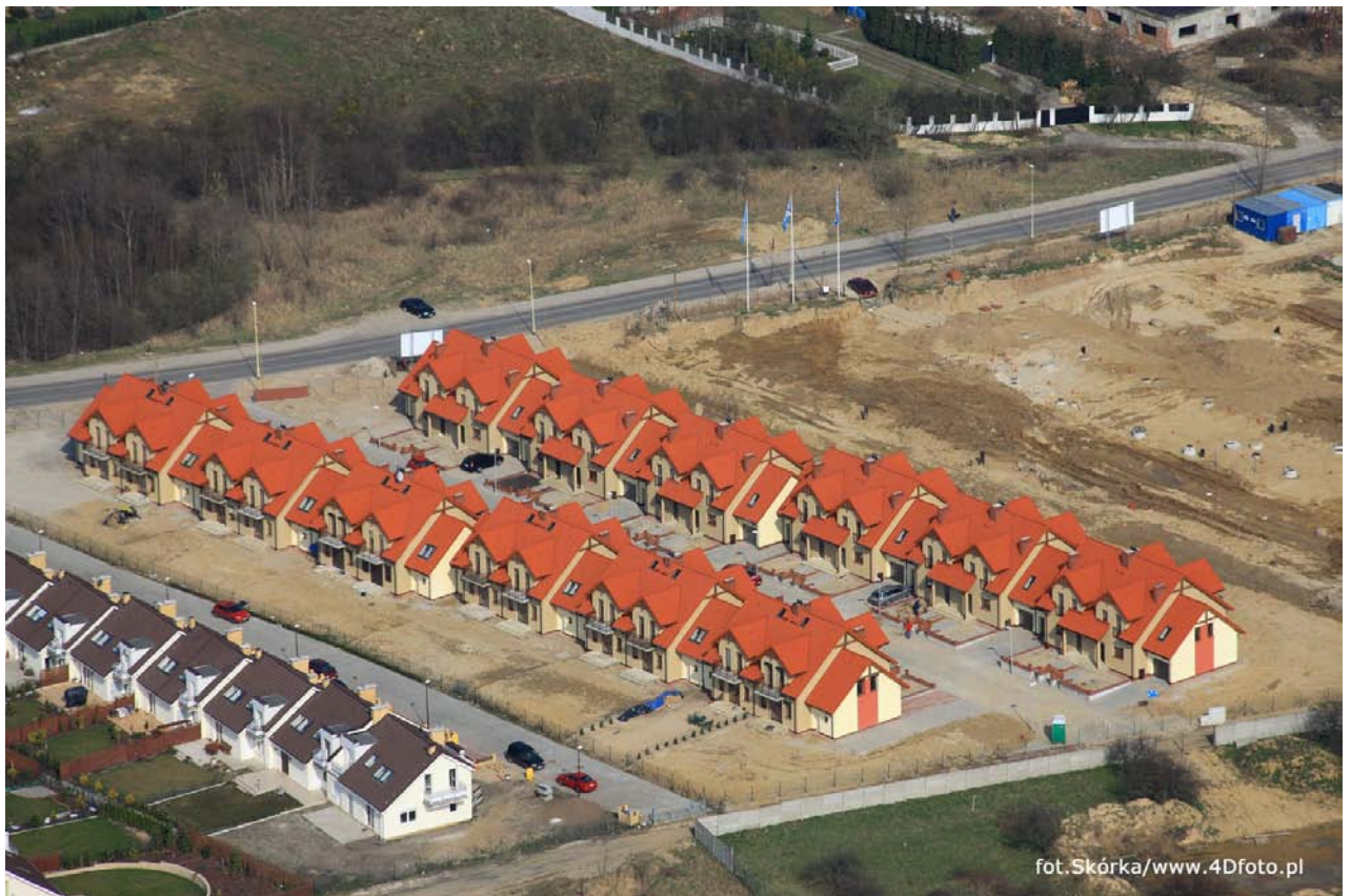
Fig. 16: The literature on sociology, psychology describes well the consequences brought by the civilisation development, the impact of the space structure in housing estates as well as natural environment on the human health. Photo: Cezary Skórka www.4Dfoto.pl .
