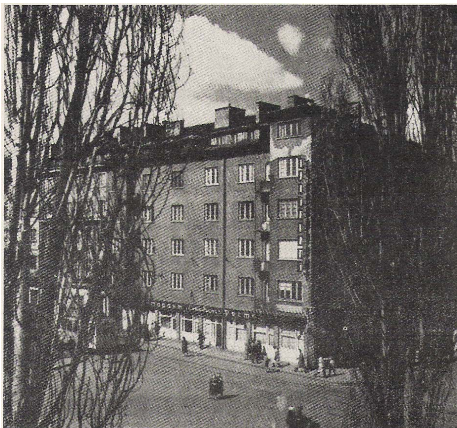
Fig.4 Graf Ignatiev multifamily residential building at the corner of Graf Ignatiev St. and Vasil Levski Blvd., Sofia 3
