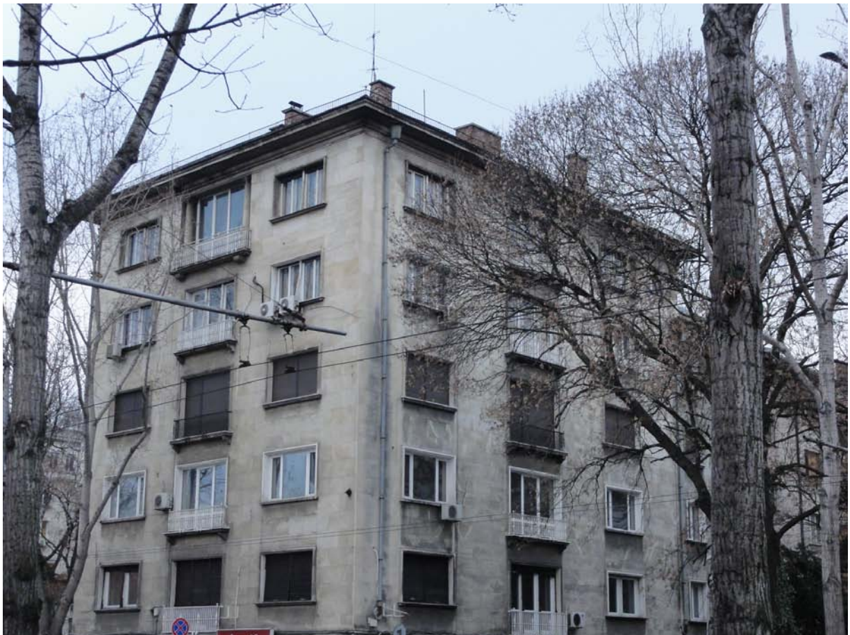
Fig. 6 Cooperative residential building at the corner of Vasil Levski Blvd. and Slavyanska St., Sofia 4
