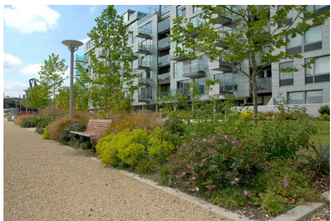
Fig. 5: Angel Waterside, Islington. All apartments benefit from external private space, either in the form of balconies , which are big enough to sit out on, or small gardens for the affordable maisonettes in the northern block.
