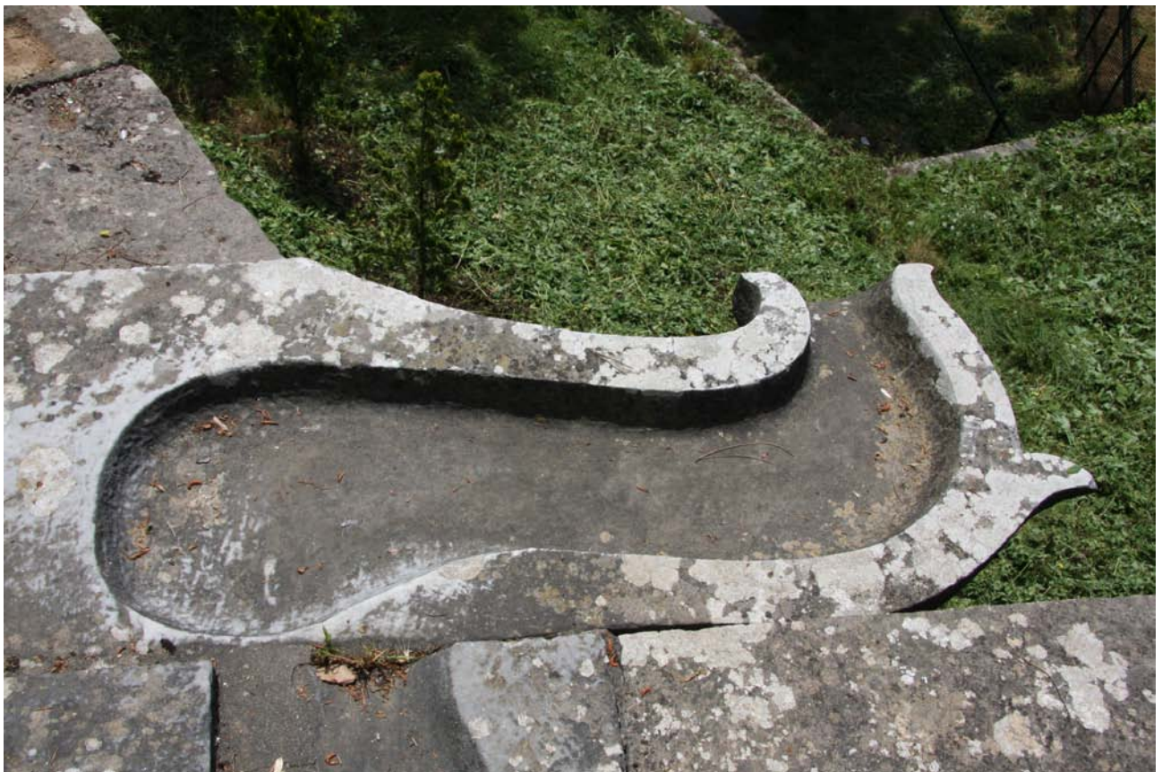
Fig. 7: The 'S' shaped gargoyles of the Sultan Mahmud II Dam
