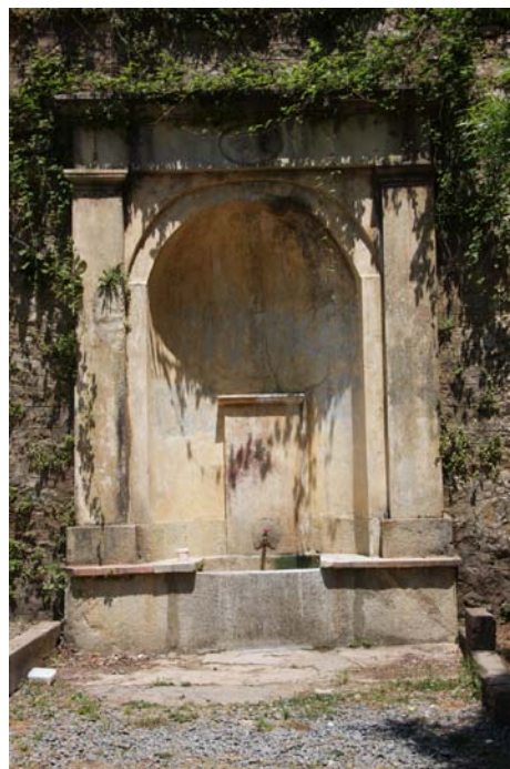
Fig. 9: The Fountain Down the Sultan Mahmud II Dam
