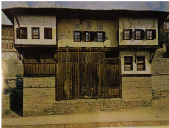
Figure 1. Kastamonu Traditional House
