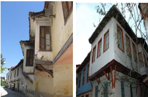
Figure 6: Old Houses in Trikala(Left) and Ioannina(Right) city cores in Greece
