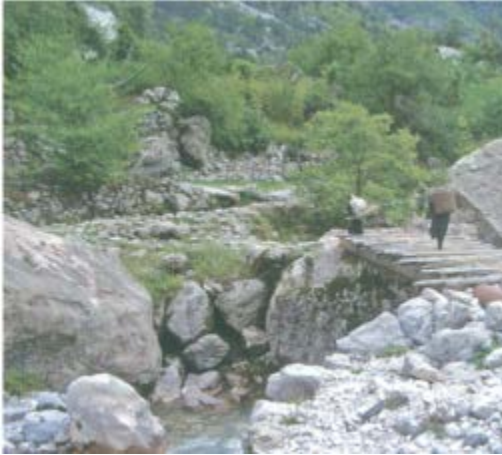
Photo 26: Bridge on the Theth Stream
