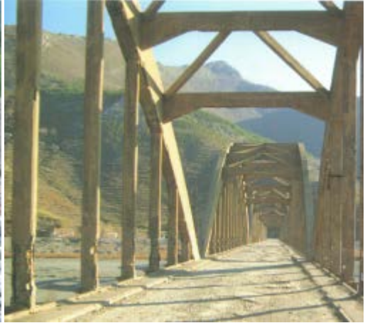
Photo 27: Ahmed Zog Bridge on the Mat Rv.
