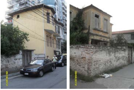
Figure 5: Old Houses in Tirana City Core(Rruga Dibres) An abandoned building in same area
