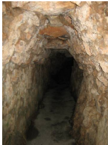
View towards inside of the tunnel (Photo: Baykan)
