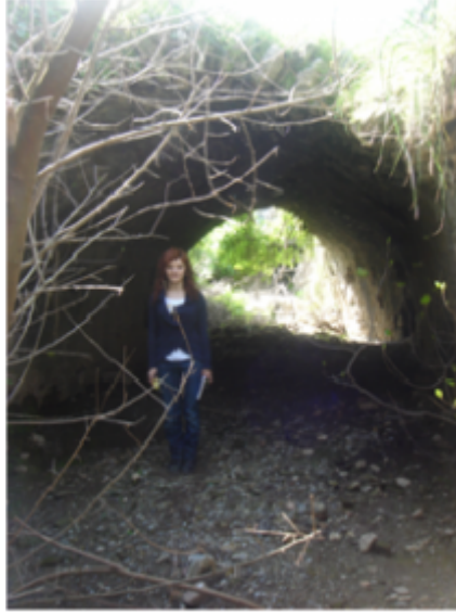
Fig. 4 Creek Covering Structure in Acarlar (Photo: A. Alkan)
