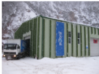
Photo 2: Plant for water packaging
