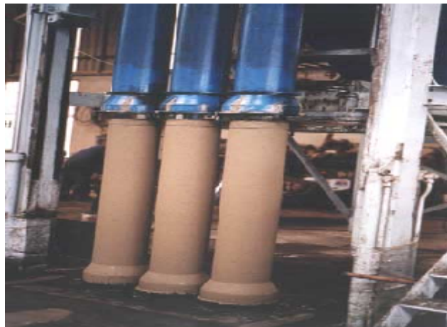
Figure 1. Specimens out of concrete pipe machine
