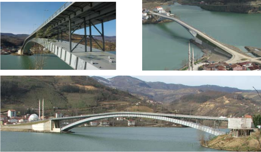
Figure 1 Some views of Eynel Highway Bridge [9]
