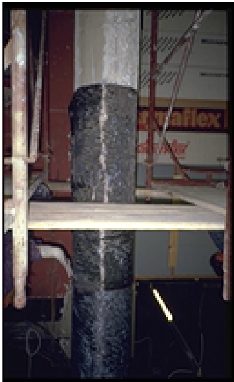
Figure 7a and 7b. The process of clothing the columns with carbon fiber texture
