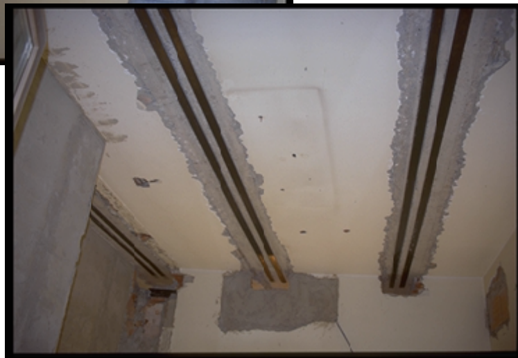
Figure 5a and 5b. The adhesion process of carbon fiber strip on the cleaned concrete surface
