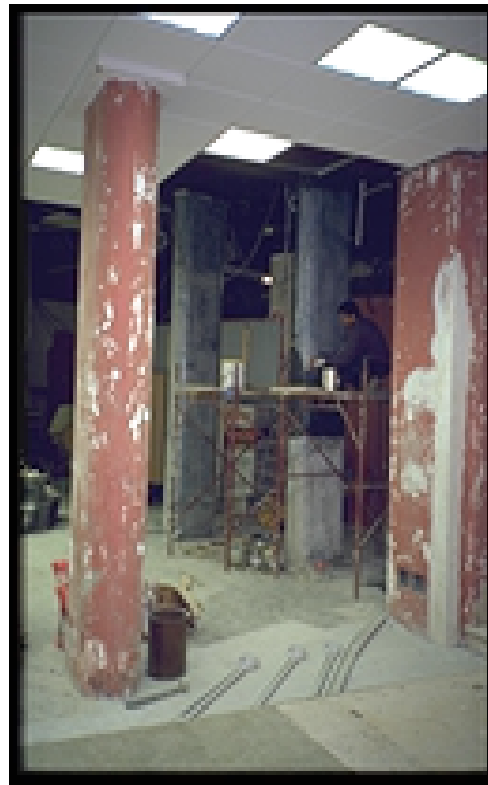
Figure 7a and 7b. The process of clothing the columns with carbon fiber texture
