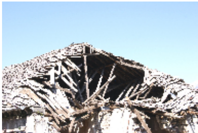
Fig. 4 Wood in roof construction
