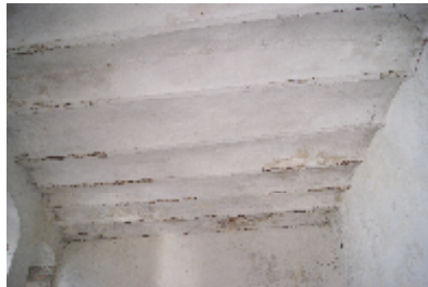
Fig.11 Brick and metal floor
