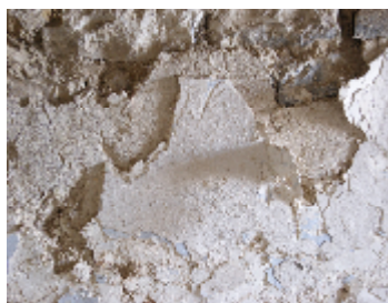
Fig. 8 Different layers of plaster
