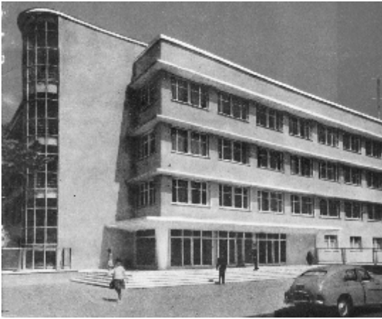
Figure 3 The Radio Building, 1967
