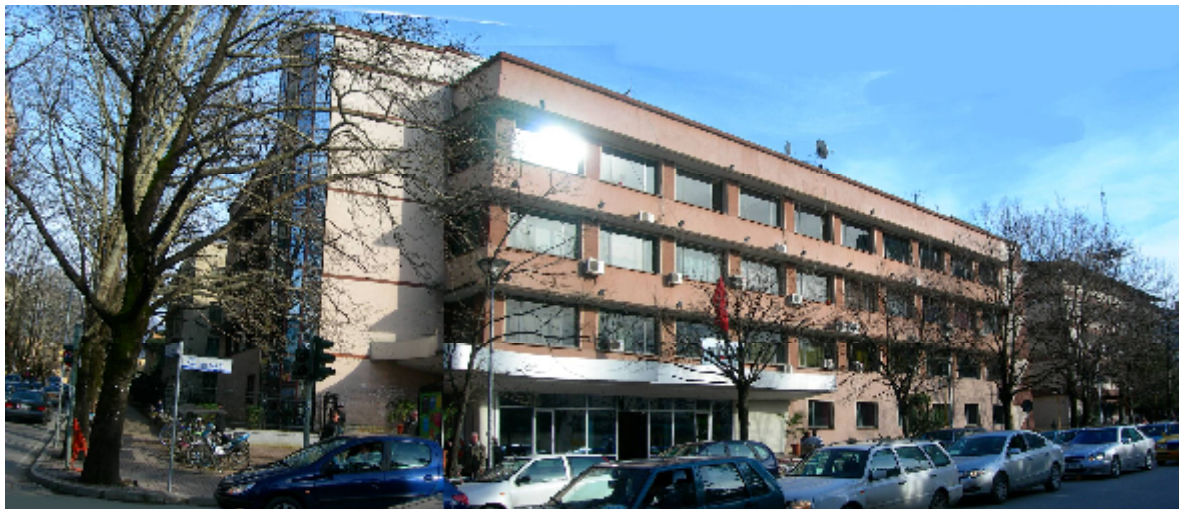
Figure 2 The Albanian RTV Complex (view of the Radio Building)
