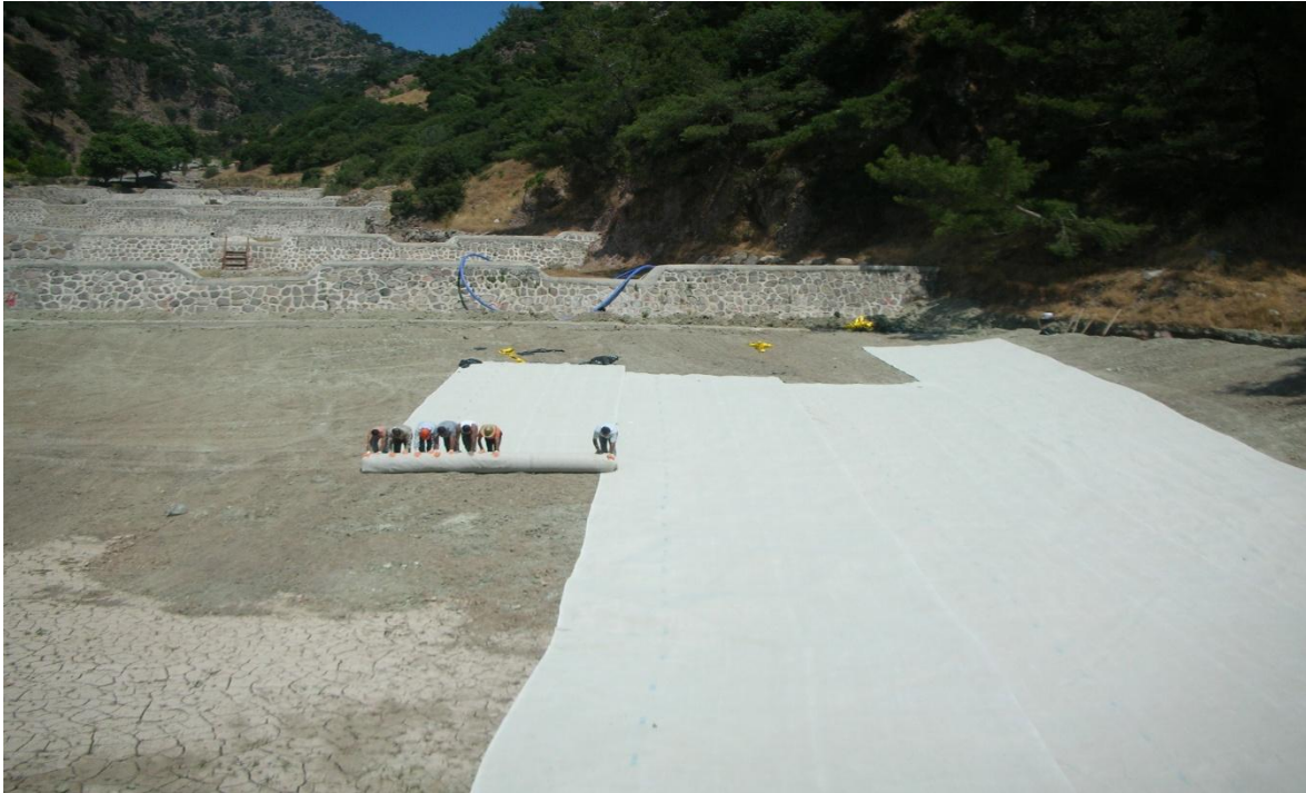
Figure 4. View of the site and Construction of GCL
