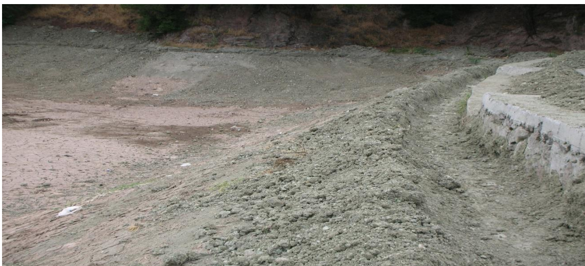
Figure 3. Trenches In The Upper Part Of The Site
