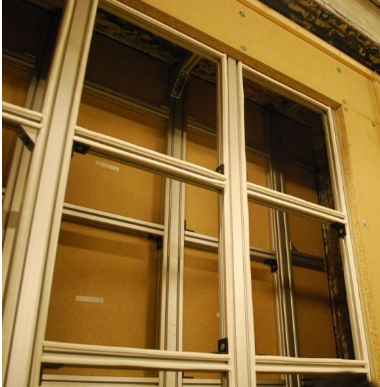
Figure 1: View of the experimental double-wall with the frame structure for the installation of flexible (individually removable) modular components
