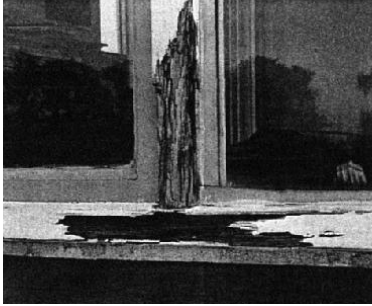
Figure 16. Wet rot and detach on wooden window (Ransom, 2005)
