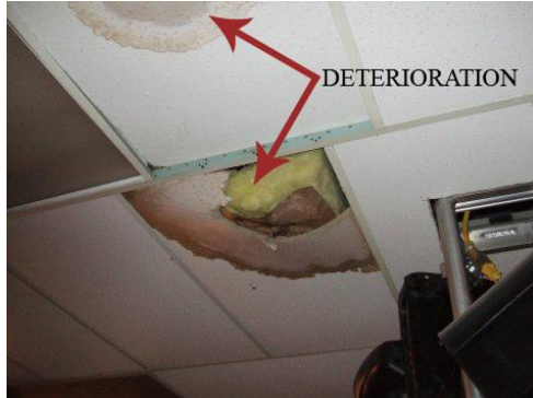
Figure 5: A building failure on installation pipes or climatization systems (Güzelçoban, 2007)
