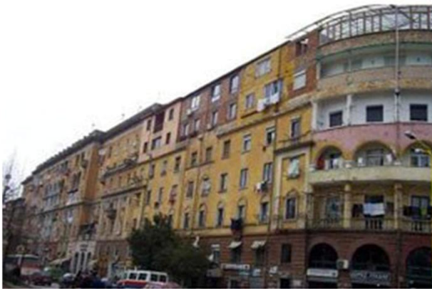
Figure 1: First division. The original facade of Shallvare's block
