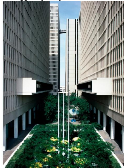
Figure 3: Site view in Atlanta, GA shows of green courtyard between the buildings
