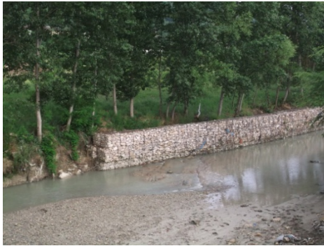
Photo 18&19: Protective measures against erosion
