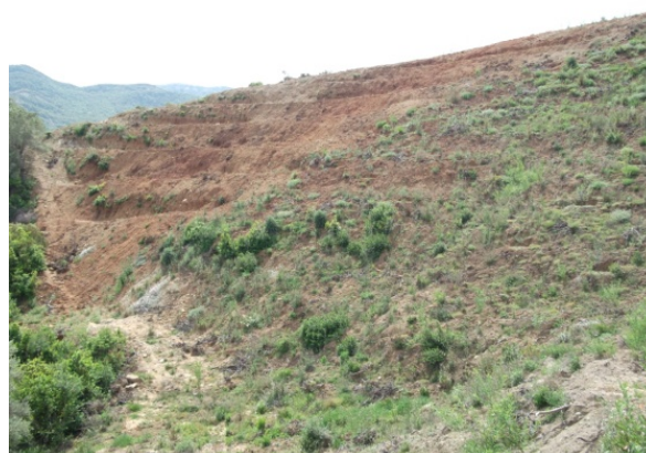
Photo 9: Digging new land accompanied with landslides(Isufmucaj 2013) Photo 10: Landslide of the created terraces (Kocaj 2013)
